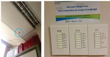
Figure 3. Photosensors close to windows and lighting switch interfaces in corridor.
